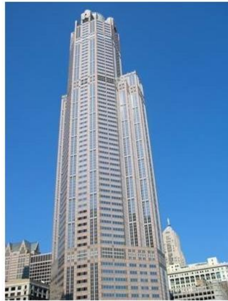
311 South Wacker Drive (1949) Chicago, 293 m, 65 storied
