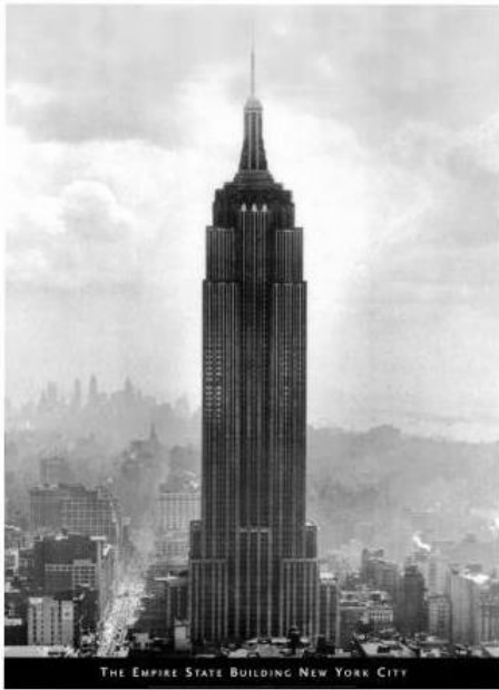
The Empire State Building (1931) New York, 381m, 102 Storied
