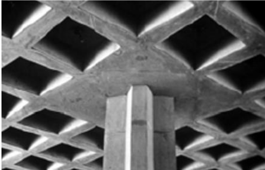
Figure 1 : waffle slab
